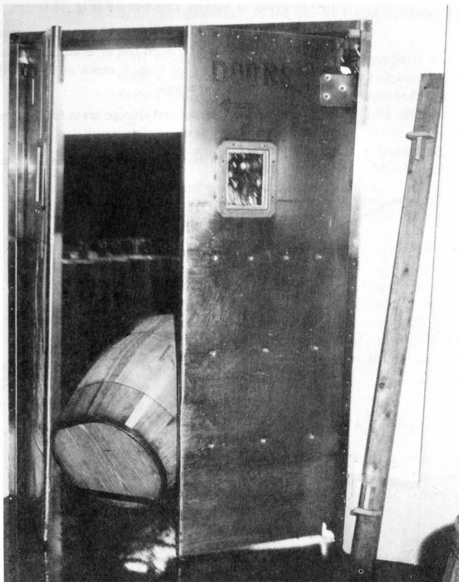
Figure 2.—Self-closing doors leading from loading platform to cooled working area help prevent temperature increase. Note doors entirely metal sheathed.
